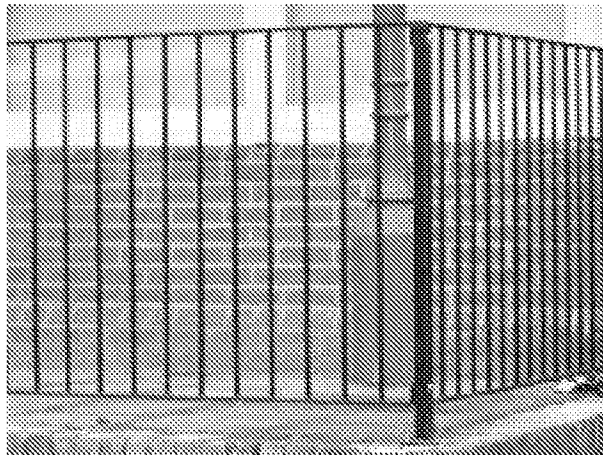
New Metal Balustrading
