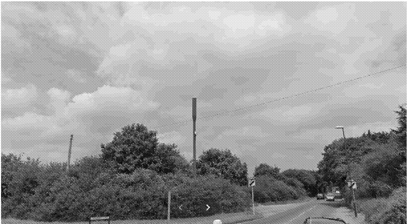
Image 1: Existing 2G/3G/4G site
