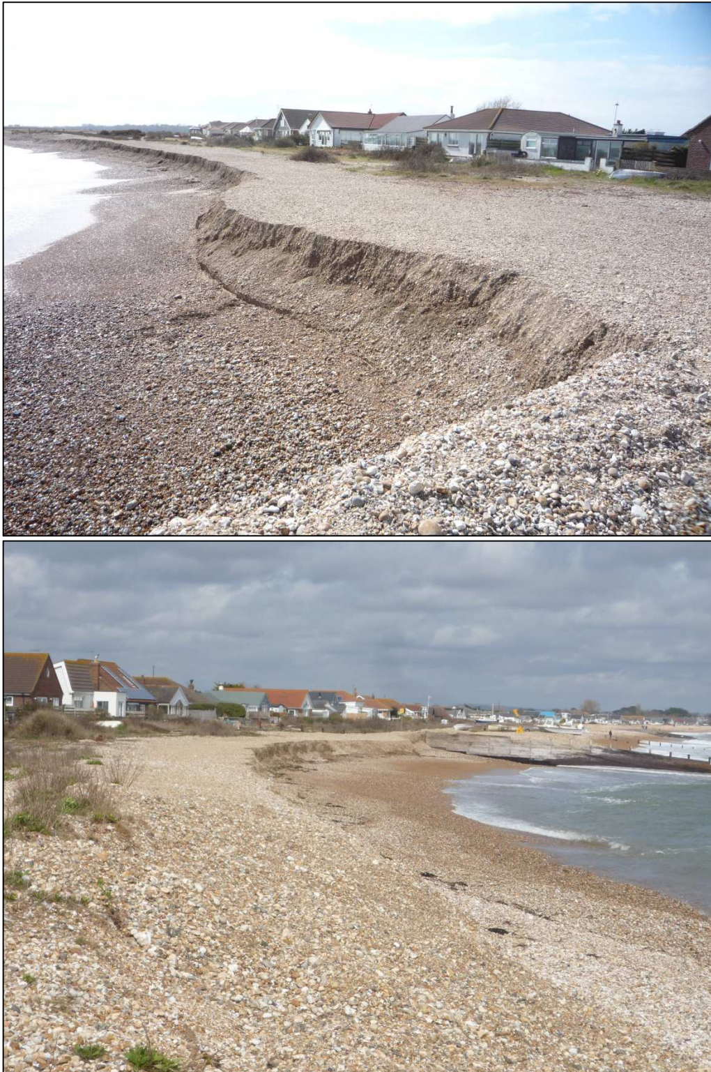
Plate 1.2: Pagham Beach frontage in 2013 following the winter storms in 2012/2013
