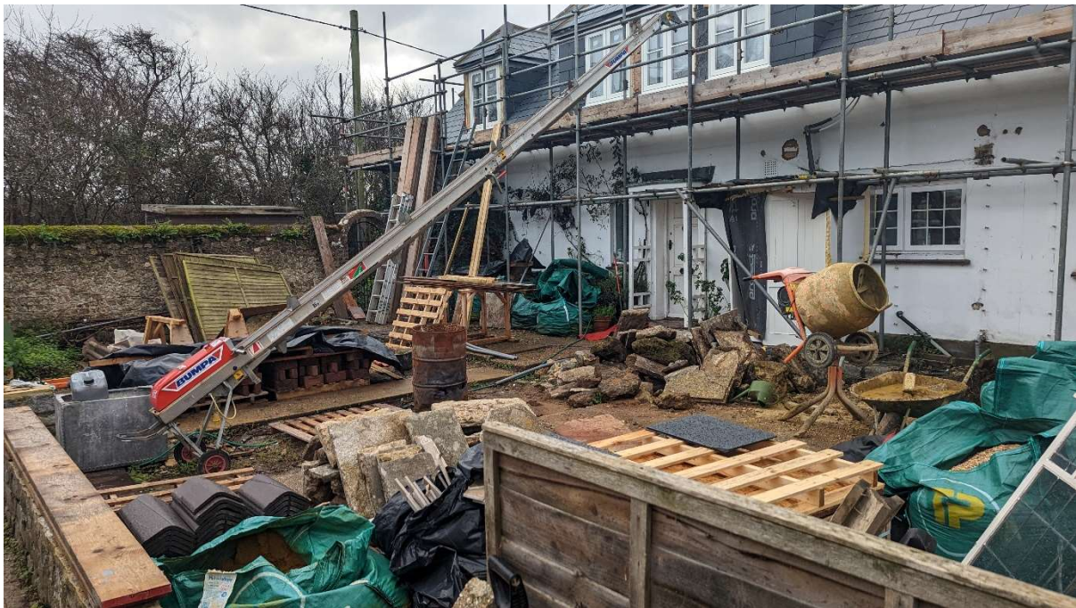
Photo 8 – View of the western hard surfaces between dwelling and garage.
