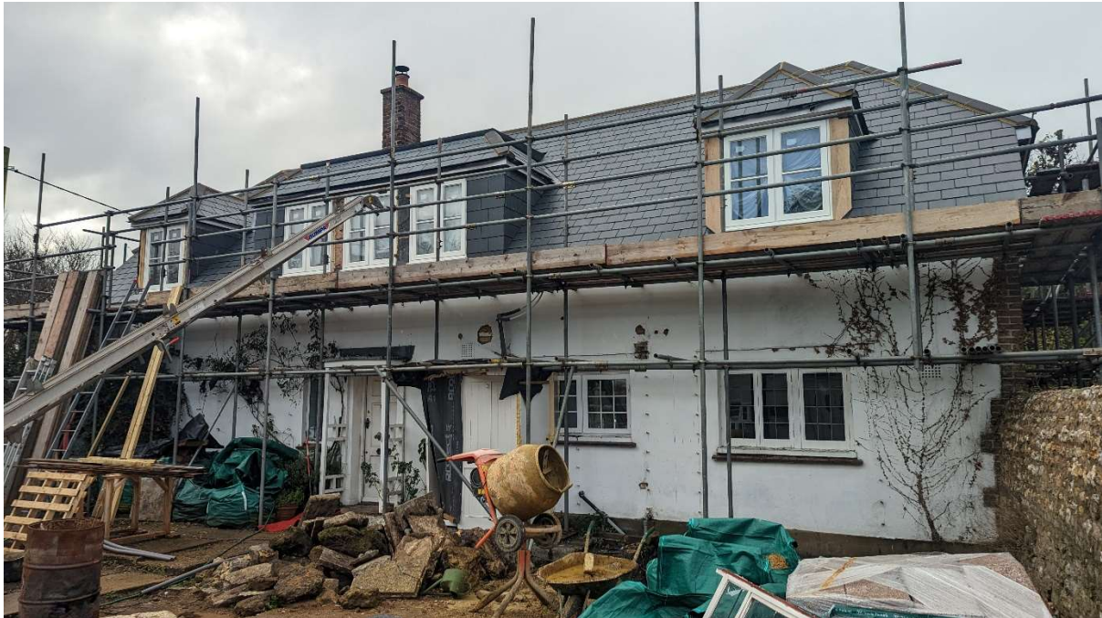
Photo 1 – View of dwelling roof from the east.
