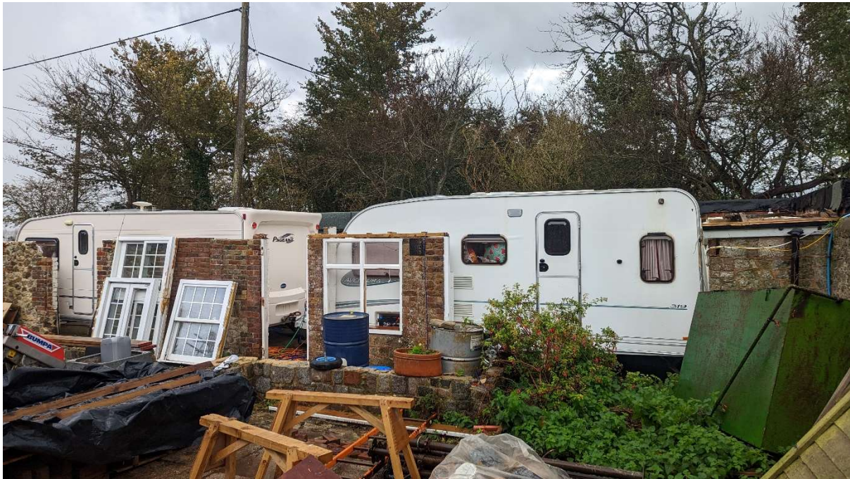
Photo 5 – View of remains of the garage, and hard surfaces between this and the dwelling.
