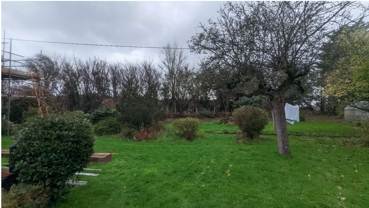
Photo 7 – View of the remains of the garage roof and door.
