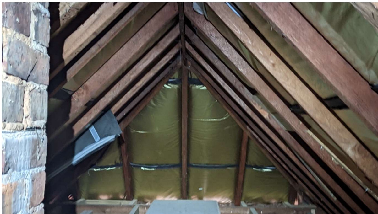
Photo 3 – View inside the loft.
