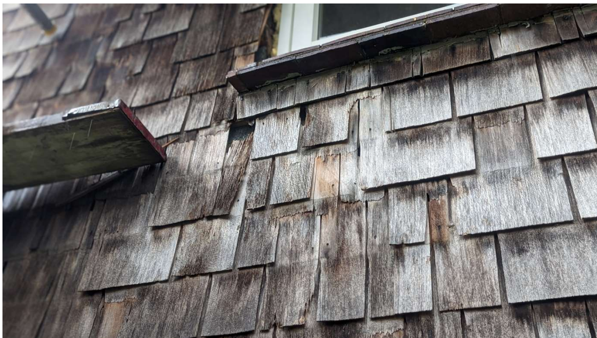
Photo 4 – View of the shingles to the south.
