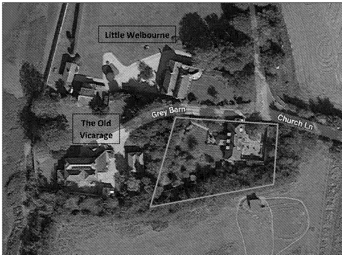
Figure I: Grey Barn (indicated by red line) in context of surroundings (Google, 2022)
