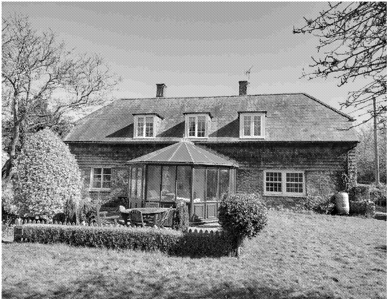
Plate I : The West Elevation of Grey Barn with PVCu Conservatory at odds with the style of the traditional barn form of the building.
