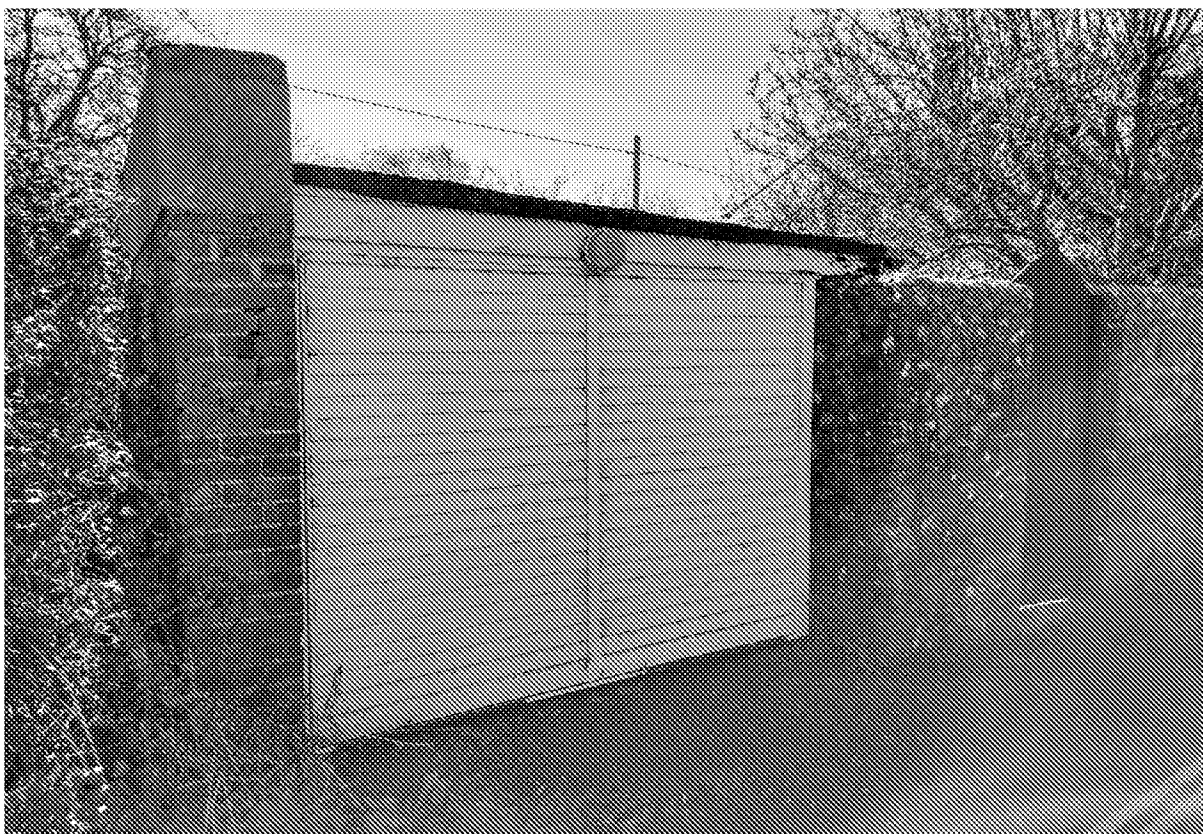
Plate VI : Grey Barn Garage – North Elevation dominated by a modern painted metal door.
