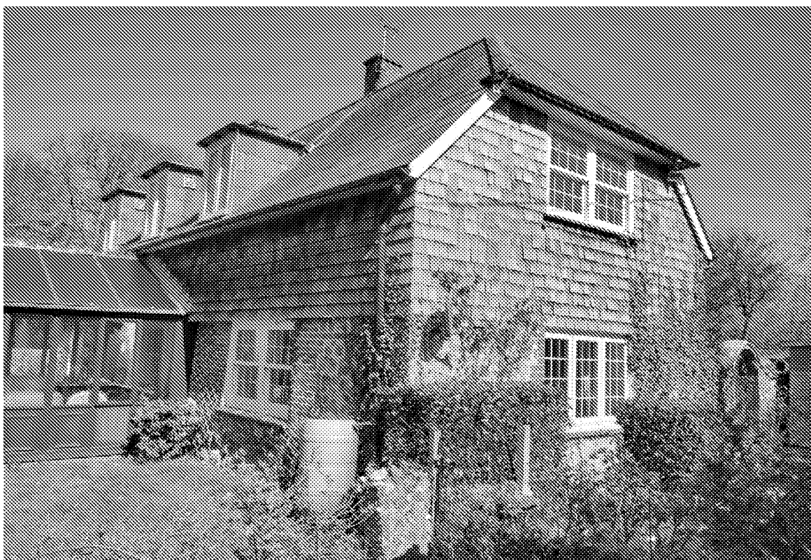
Plate II : Grey Barn – South-west perspective. The white PVCu windows at odds with the muted, natural tones of the shingles and roof slates.
