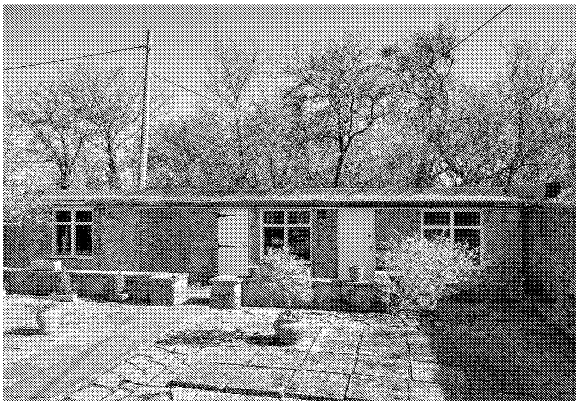
Plate V : Grey Barn Garage and ancillary store – West Elevation into concrete covered courtyard.
