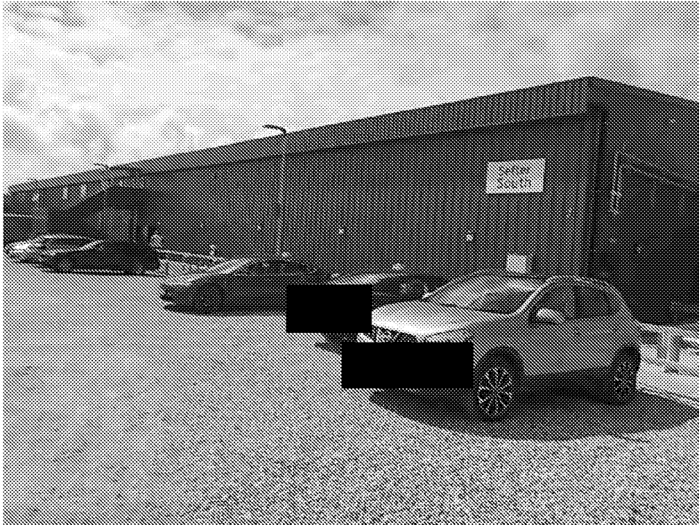
View on existing car park
