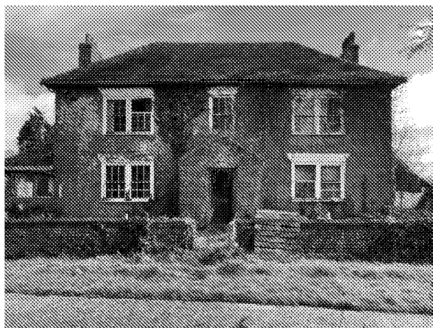
Figure 2 - The front (west) elevation with entrance porch
