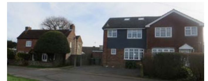
Hook Lane - Irregular Frontage
