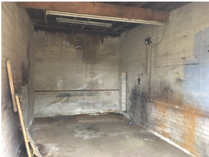
Figure 2. Internals of one of the garages (19/03/2018).
