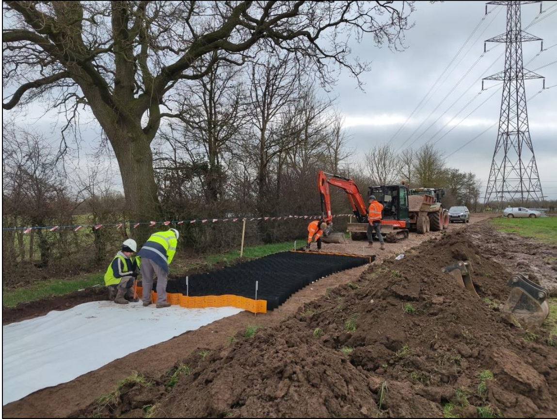
Figure A: An example of a cellular confinement system being laid.
