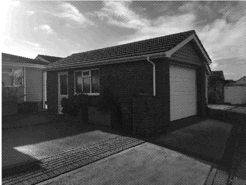
Figure i. Detached single garage at 47 West Front Road
