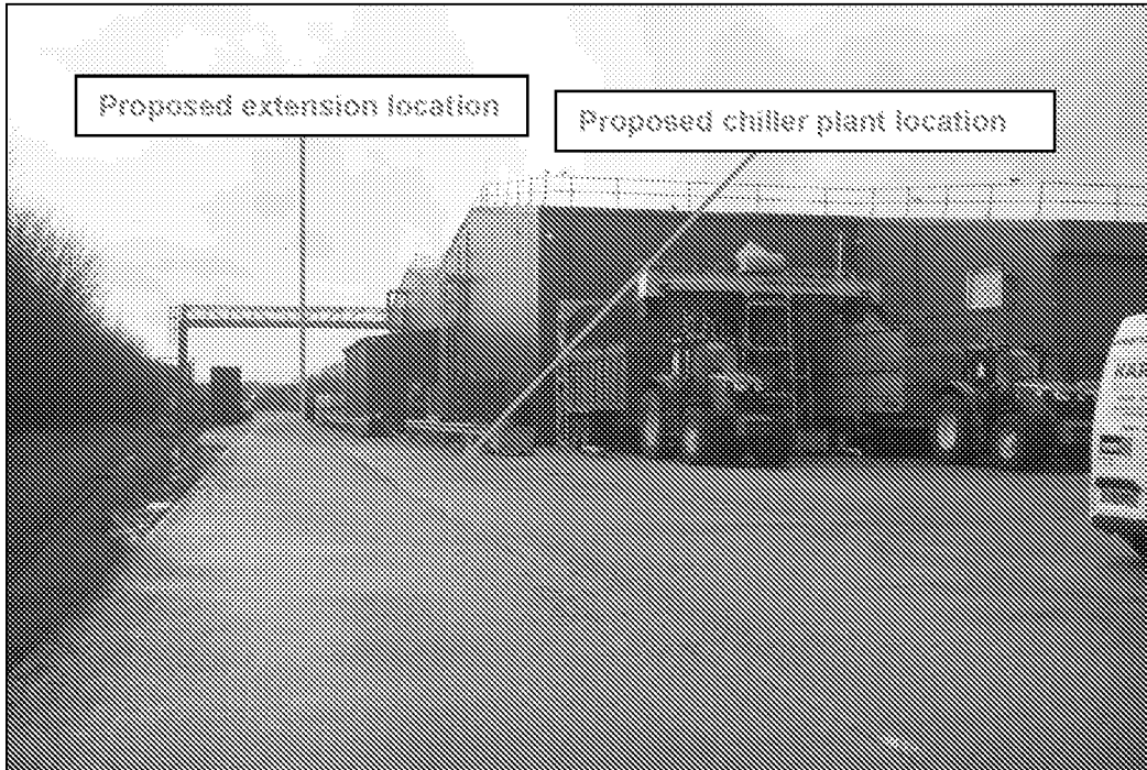
Photograph 1 Showing the proposed extension and chiller plant location
