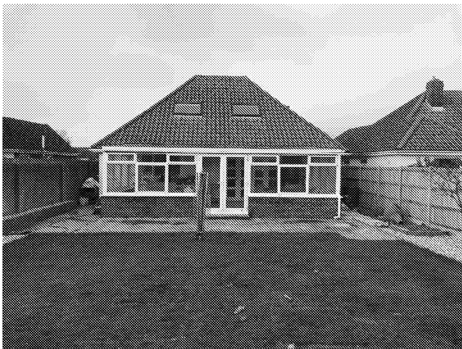
Photograph 1: South facing rear elevation of existing conservatory.
