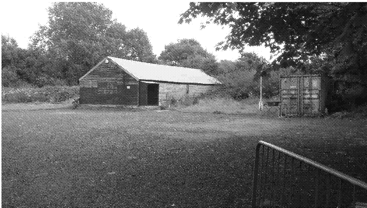
Plate 1 View of the hall in southwest corner of site, facing northeast
