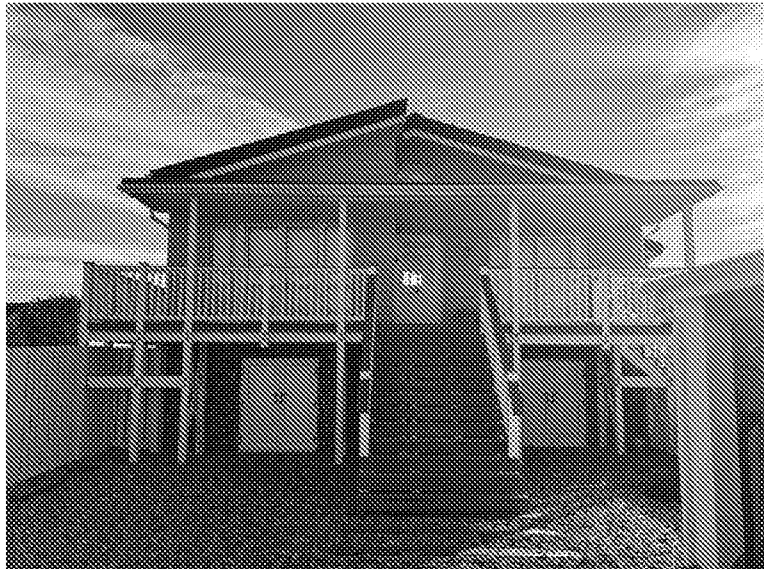
Existing Timber structures on Pagham sea front
