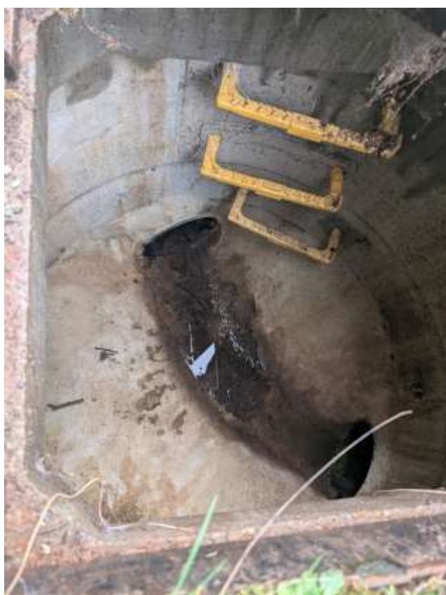
Fig 5. Existing manhole/Culvert and existing watercourse.
