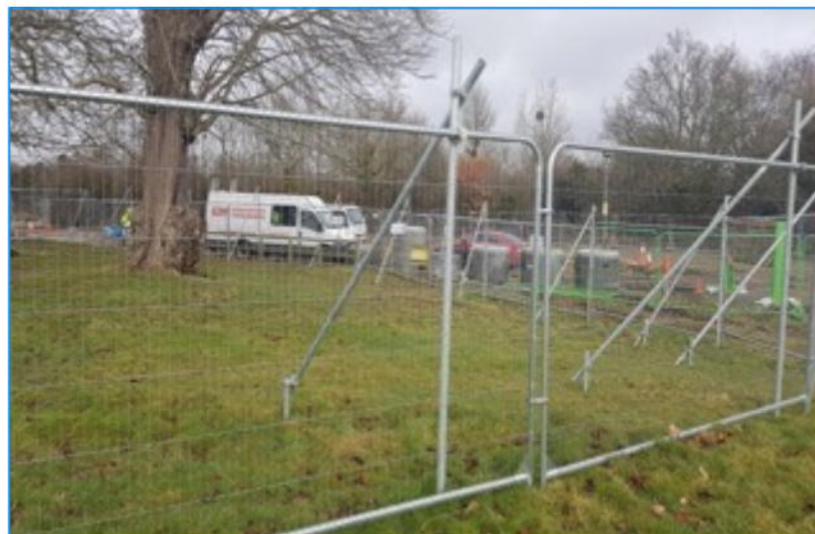
TPF 2: Alternative fencing option: scaffold uprights with backstay
