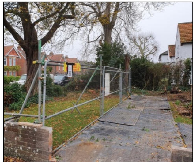
GP2: Tree protection barriers & trackmat ground protection
