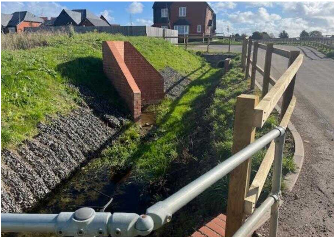
Existing culvert that is crossed twice by the new access road via Summer Lane
