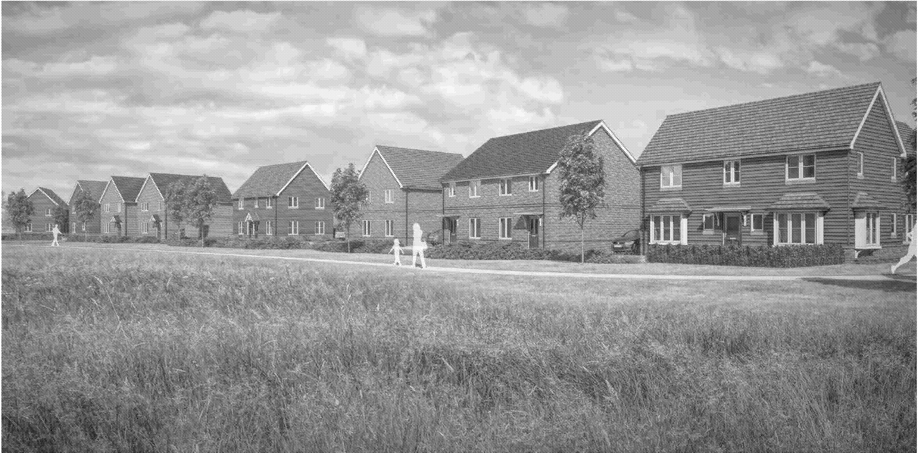
FIGURE 5.18: VIEW OF PLOTS 262 TO 269 - NORTH-WEST CORNER
