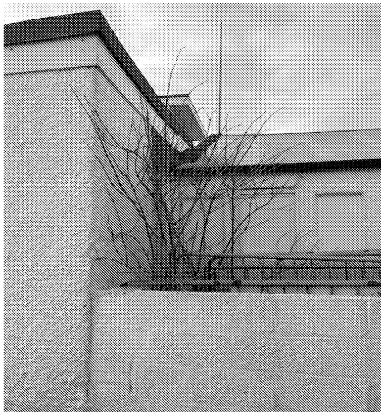
Photo 12 – Self-sown sapling abutting the building on east side
