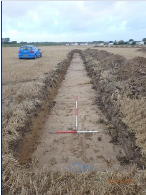
Plate 34: Trench 15, from the south-east
