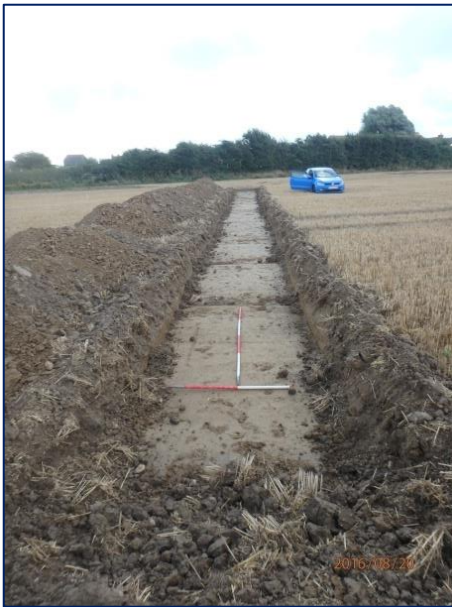
Plate 42: Trench 18, from the north-west
