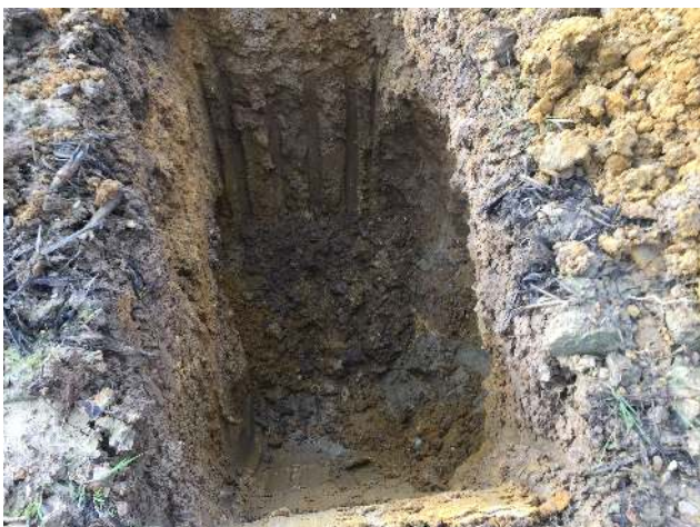
Photo 79: Excavation of trial pit IT43.
