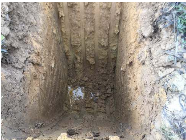
Photo 75: Excavation of trial pit IT41.
