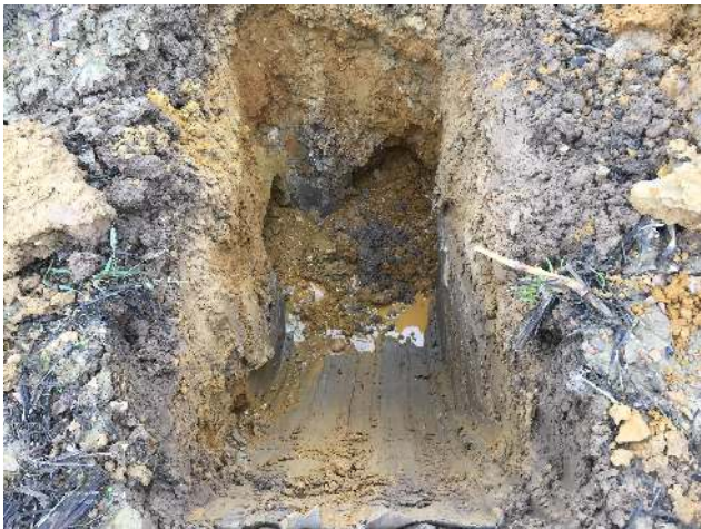
Photo 77: Excavation of trial pit IT42.
