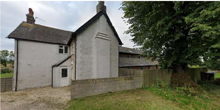
Existing White painted Farmhouse with adjacent former barn buildings that have been converted into residential accommodation at the junction of Pagam Road and Sefter Road.
