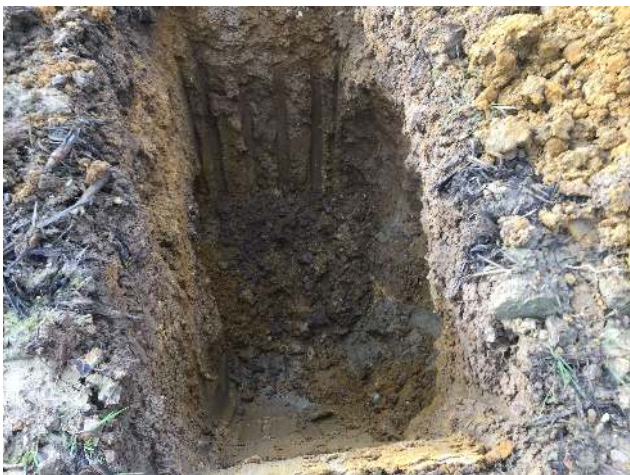
Photo 79: Excavation of trial pit IT43.
