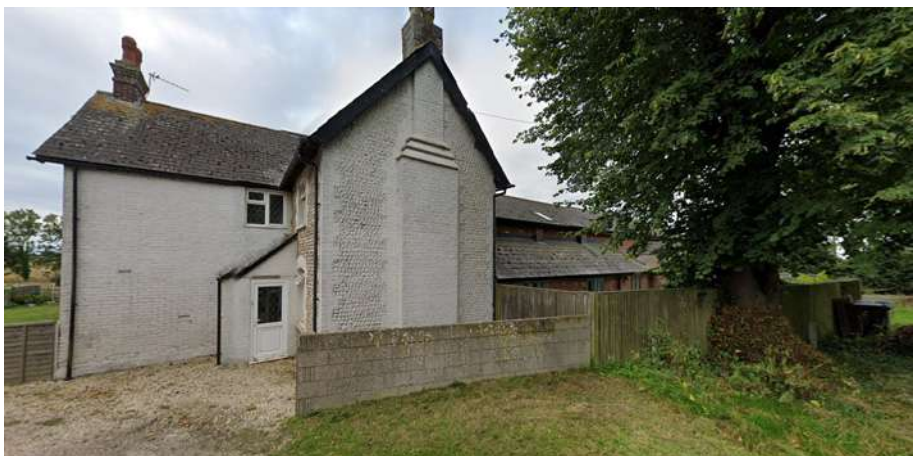
Existing White painted Farmhouse with adjacent former barn buildings that have been converted into residential accommodation at the junction of Pagam Road and Seftor Road.
