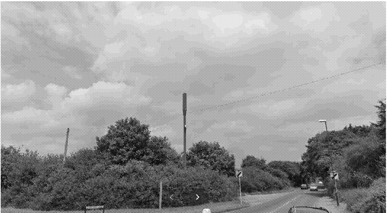
Image 1: Existing 2G/3G/4G site
