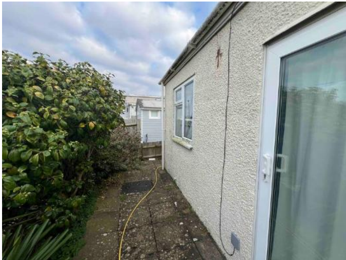
Figure 8 - view northeast to 11A West Front Road from existing platform/terrace
