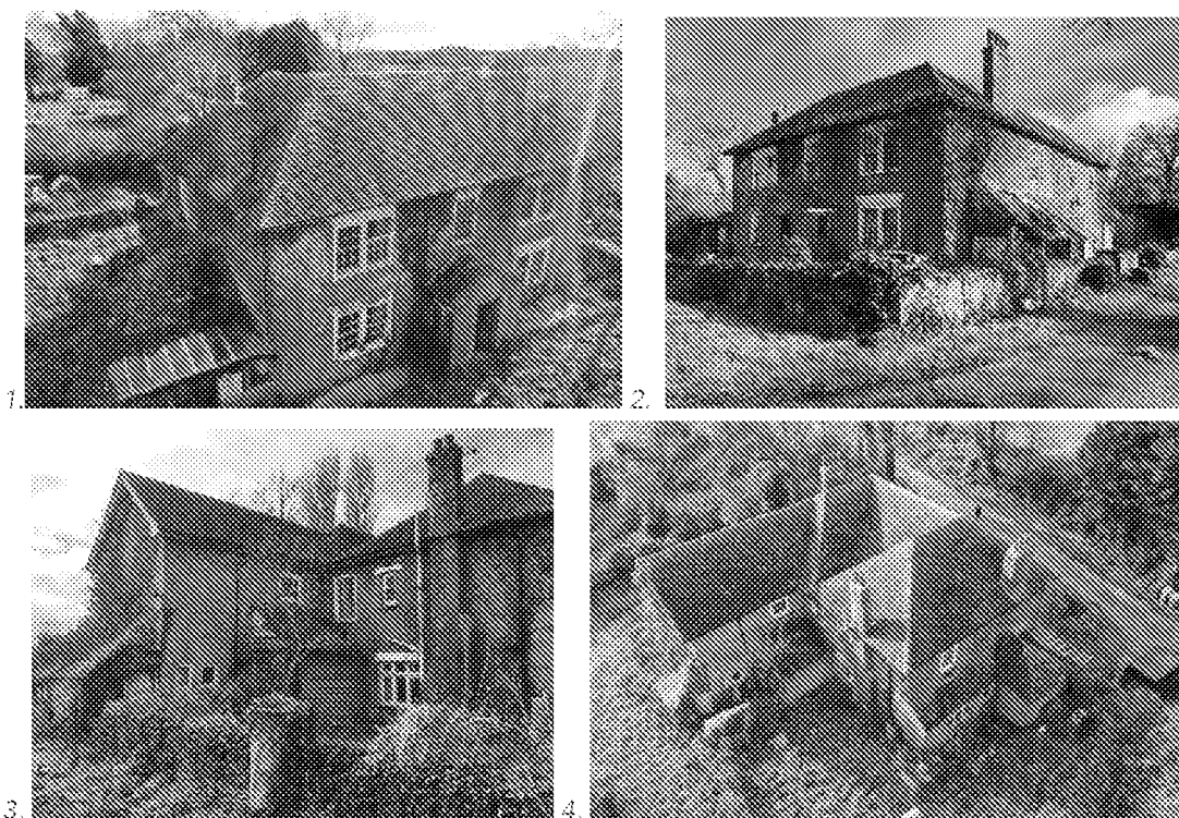
Figure 3 - 1. front/northern elevation, 2. front/southern elevation, 3. inner corner, 4. aerial view of rear
