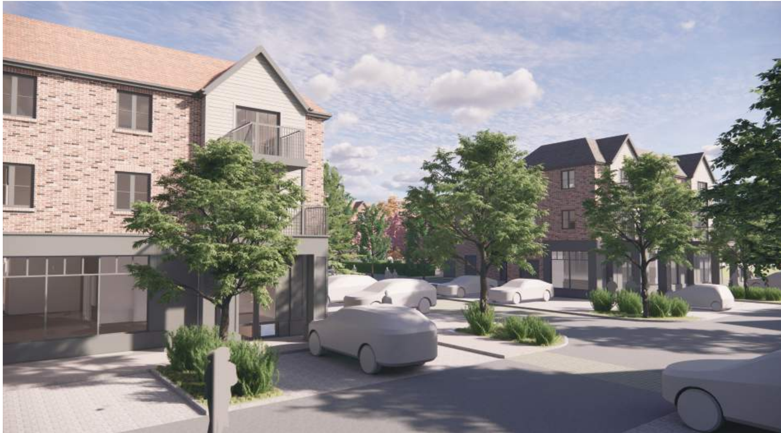
View towards block C and B from North West
