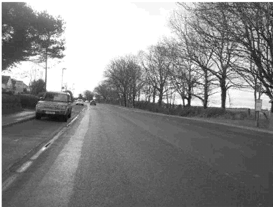
Looking south on Pagham Road. The new spine road will be to the right past the bus stop layby
