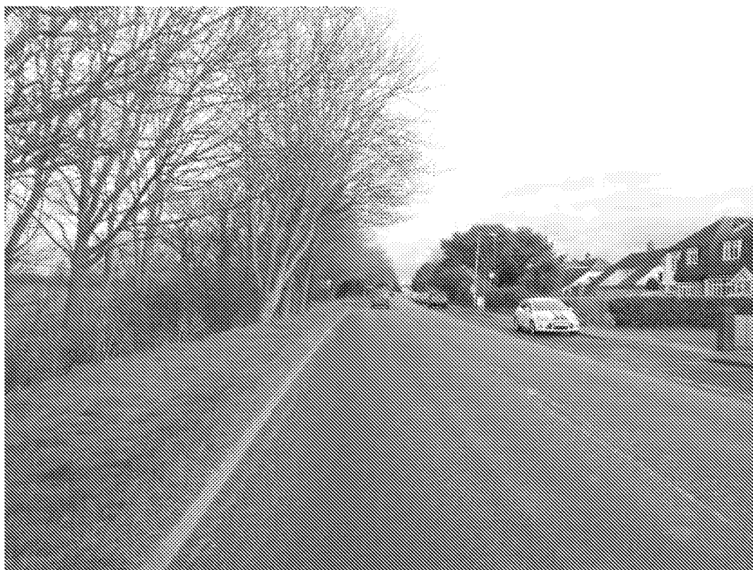
Looking north on Pagham Road. The new spine road will be to the left opposite the white car
