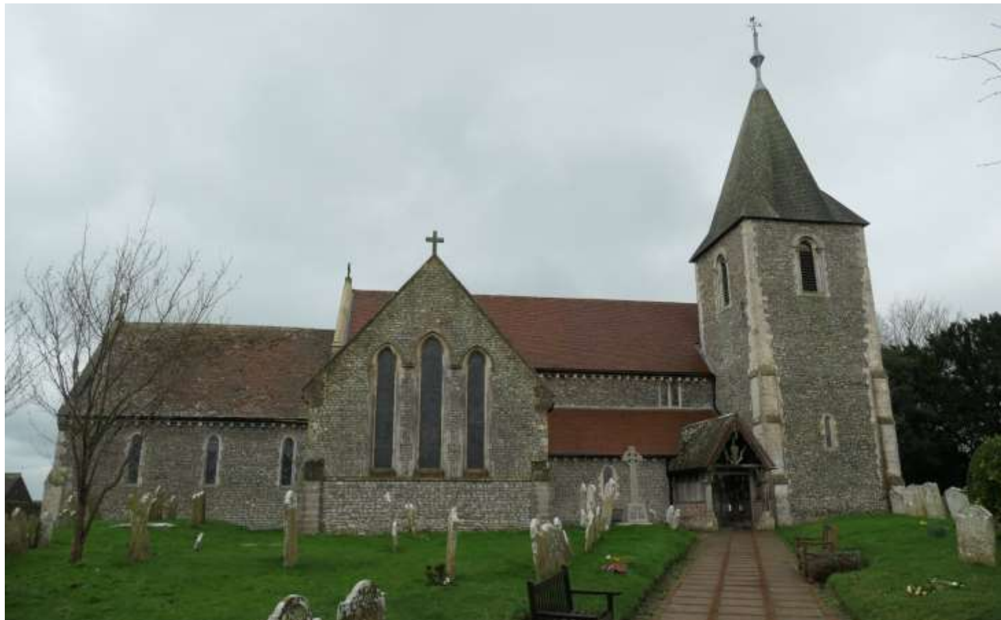
Photo 1: A close frontal view of the church from the north.
