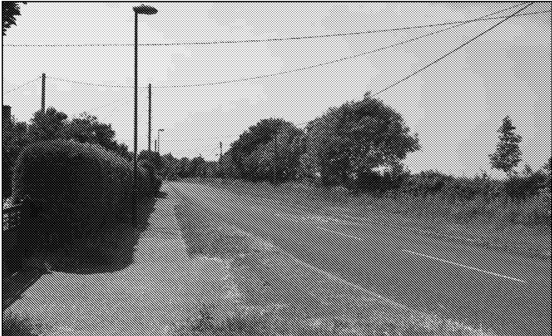
Photograph 4 – view south on Pagham Road, looking towards the proposed southern access from the opposite side of the road
