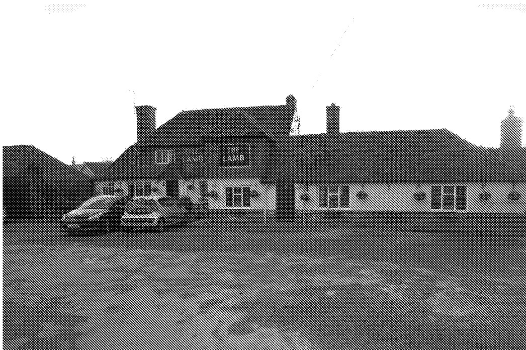
Pl.23: The Lamb, Nyetimber, from the north.
