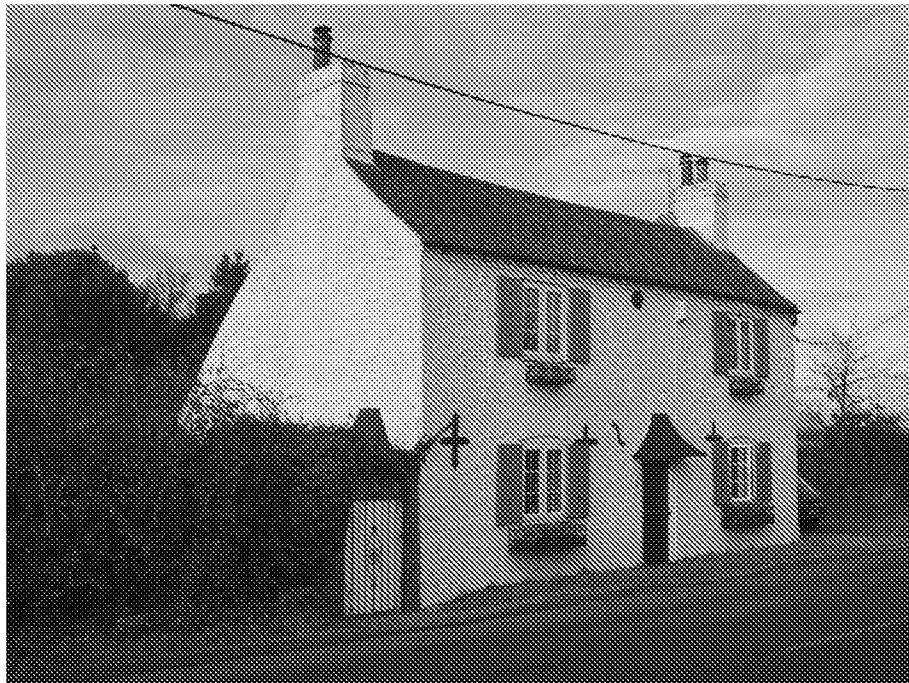
Pl.24: No.25 Pagham Road from the south-west.
