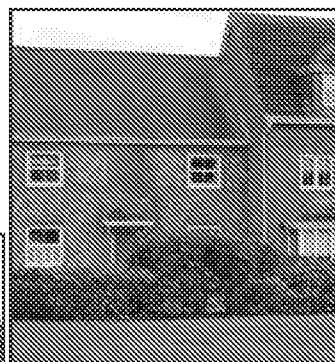
BRICK QUOIN DETAILS AROUND THE WINDOWS AND EDGE OF BUILDINGS
