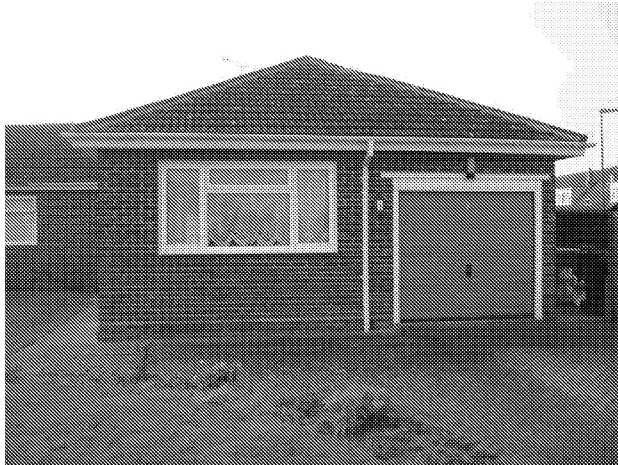
Photograph 1. Front elevation of the existing garage (north east elevation).
