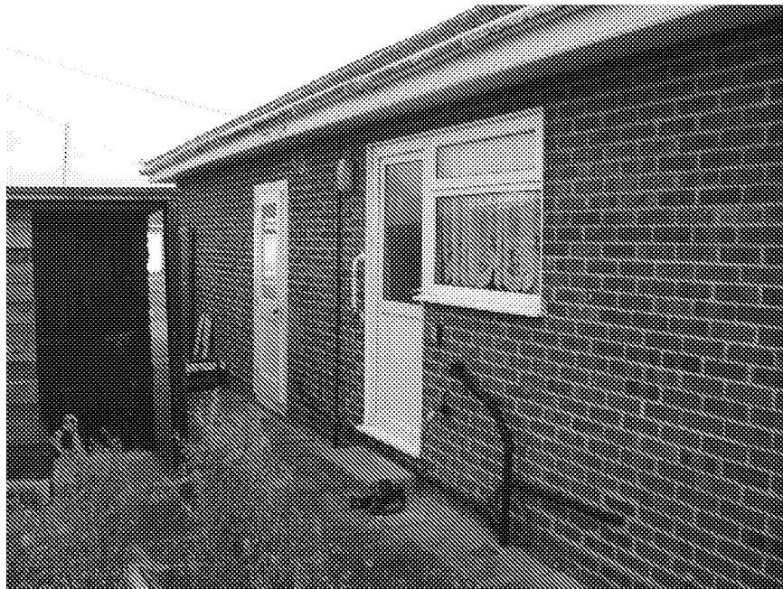
Photograph 2. Side elevation of the garage. Note the single timber door on the far left of the picture provides access into the garage. The single uPVC door on the right of picture will be removed and bricked up. (north west elevation).
