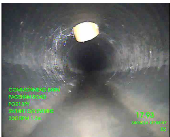
c8d445c6-5c97-4394-a9b1-9c6aadde0601.jpg, 00:01:34, 17.93 m Connection other than junction at 12 o'clock, 100mm dia
