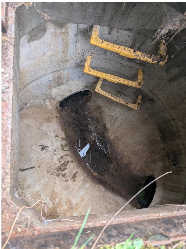
Fig 3. Existing manhole/Culvert and existing watercourse.
