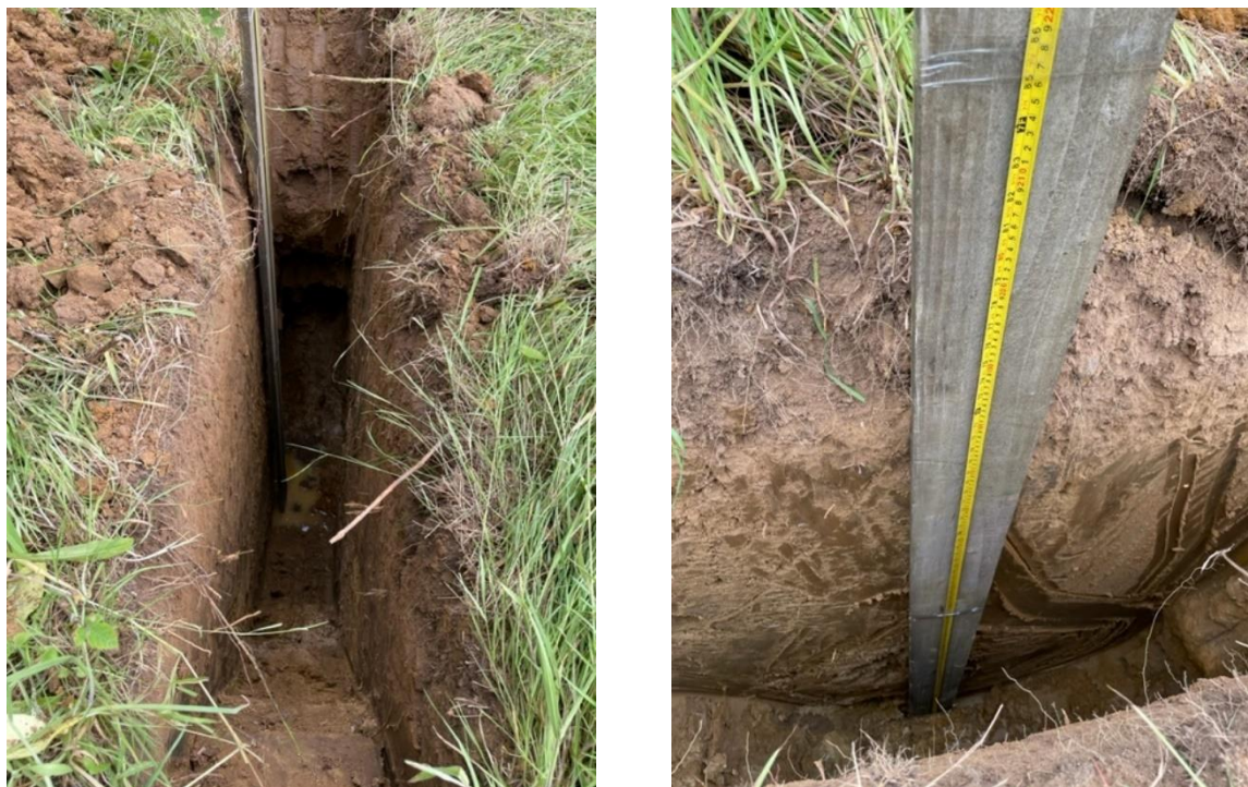
Fig 3. Soakaway test photographs
