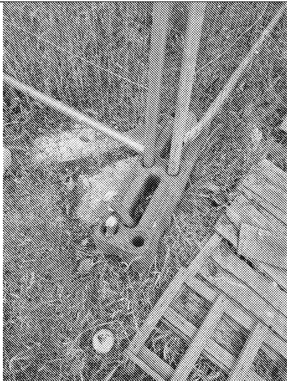
Picture 5 – Example of how fencing feet have been pinned in to location, these lengths are c.40cm long
