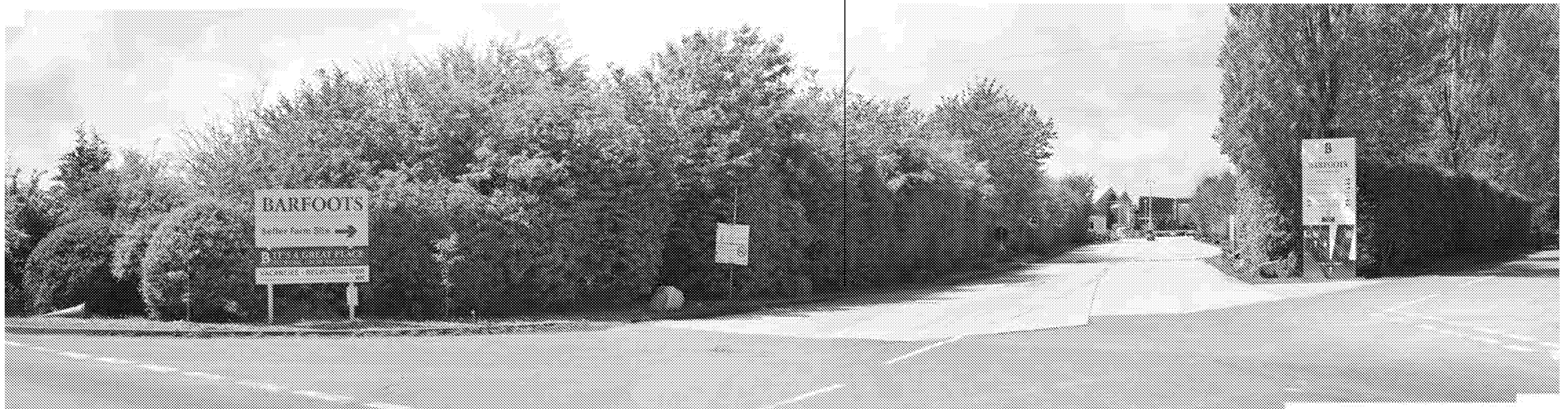
Panoramic view from Pagham Road looking west into the site at the entrance to Seifer Farm
