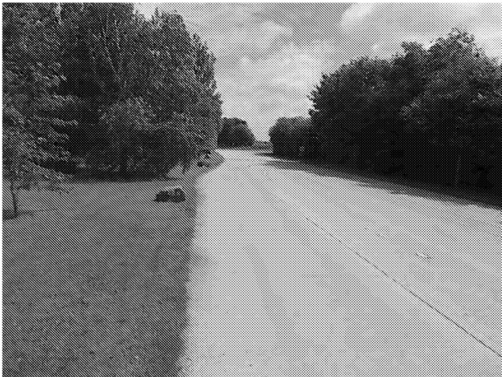
View on existing access road
