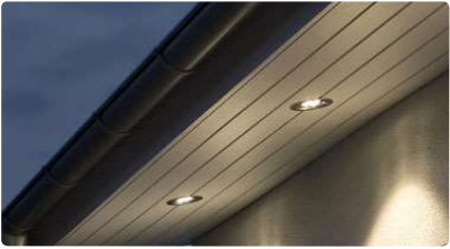
SOFFIT & EAVES LIGHTING
