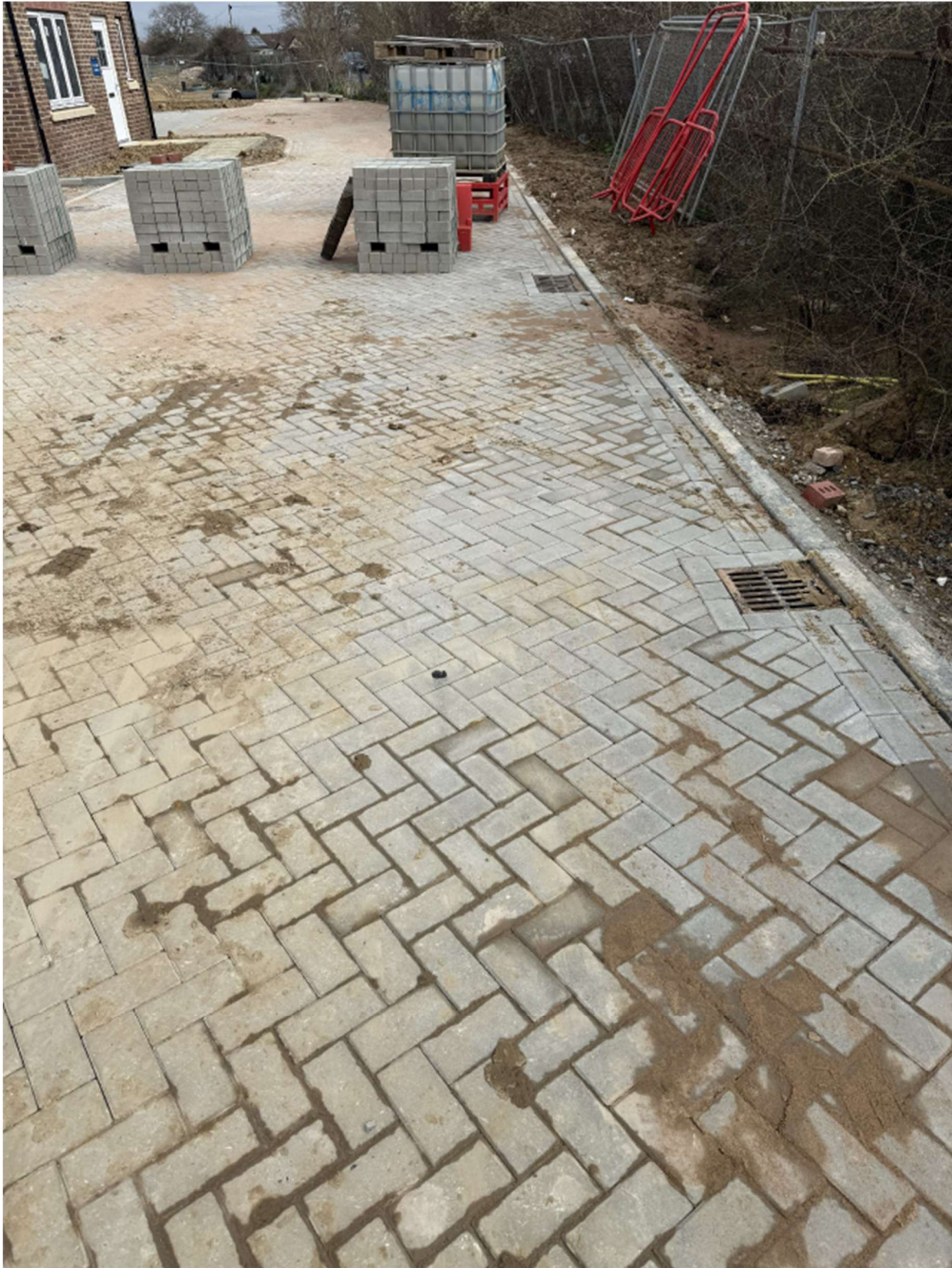
Figure 11 – Road gullies in access road outside Plot 268
