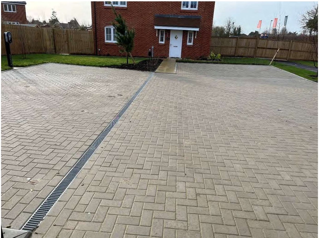
Figure 2 - Drainage channel within plot 12/13 parking area
