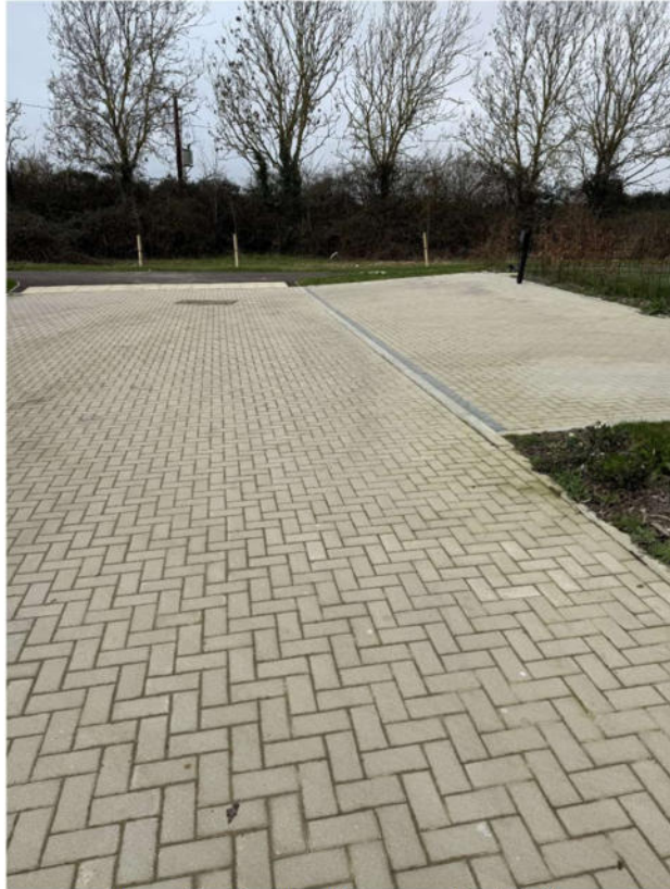
Figure 7 – Road gullies opposite plot 31
