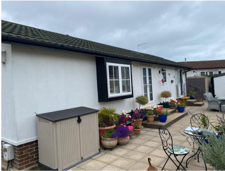
Photo 3 to show: Existing rear elevation (West).
