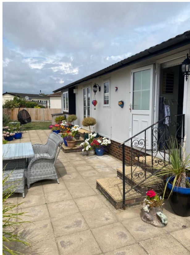
Photo 4 to show: The rear elevation and the southern end where the steps to the single external door to the kitchen are to be demolished and where the position of the new conservatory is proposed.
