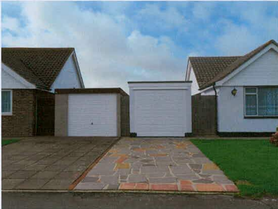
Photo 8 Garage to be demolished and No24
