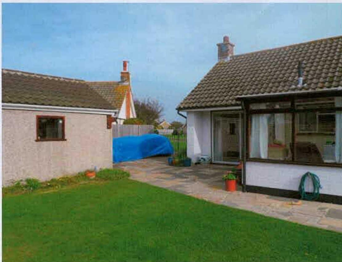
Photo 5 Conservatory and garage
