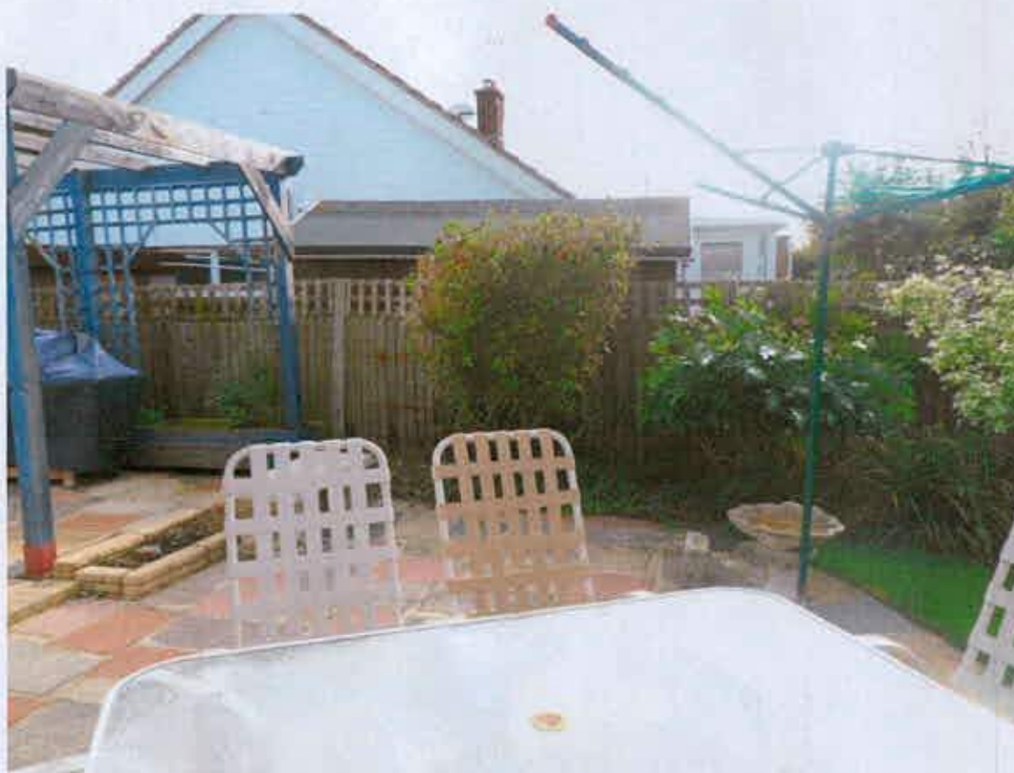
Photo 6 North (Side) elevation of No 24 Leonora Drive
