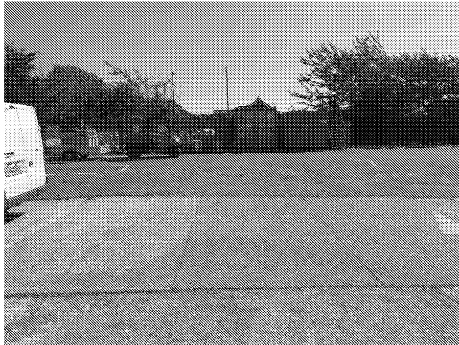
External Photograph of the existing Maintenance Yard
