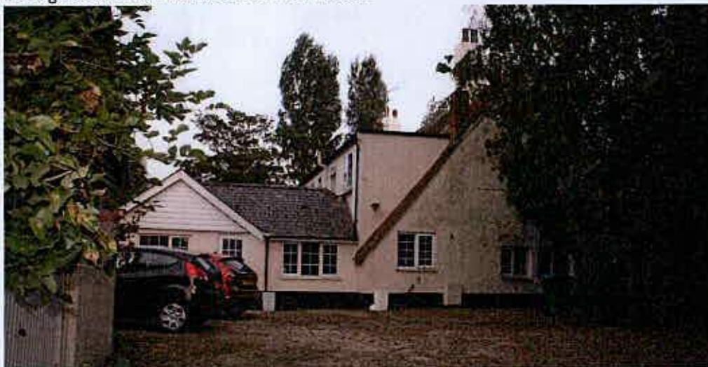
Photo: Hostel car parking West end of Sefter Granary, looking East, taken from within the garden.
