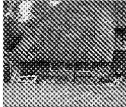
Southern outshot to be altered (left) and 16 th century mullioned window to be exposed (right).
