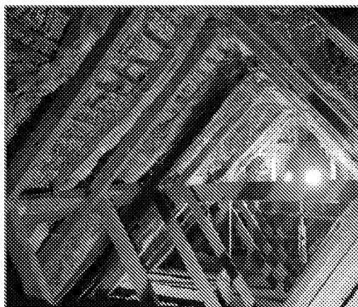
Roof structure with 1970s supportive structure.
