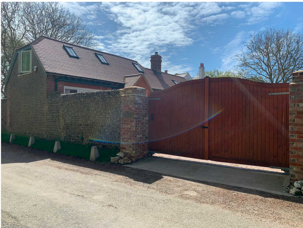
View from Poling street looking towards north and west elevations of the existing property
