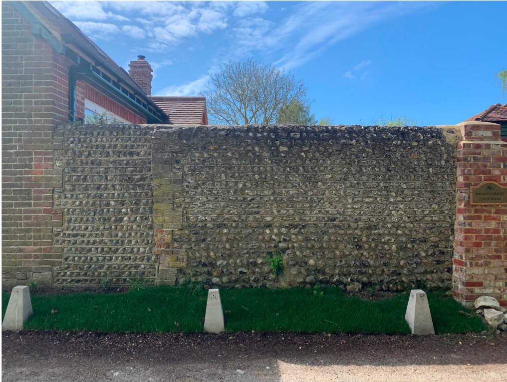
View from Poling street towards south
